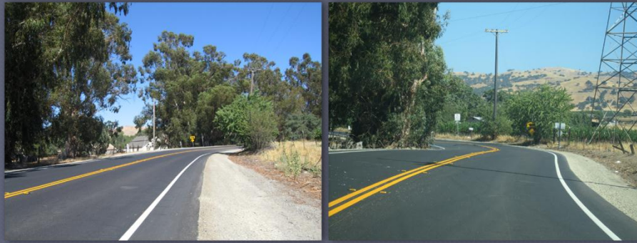
Realigned Curves to Increase Sight Distance
